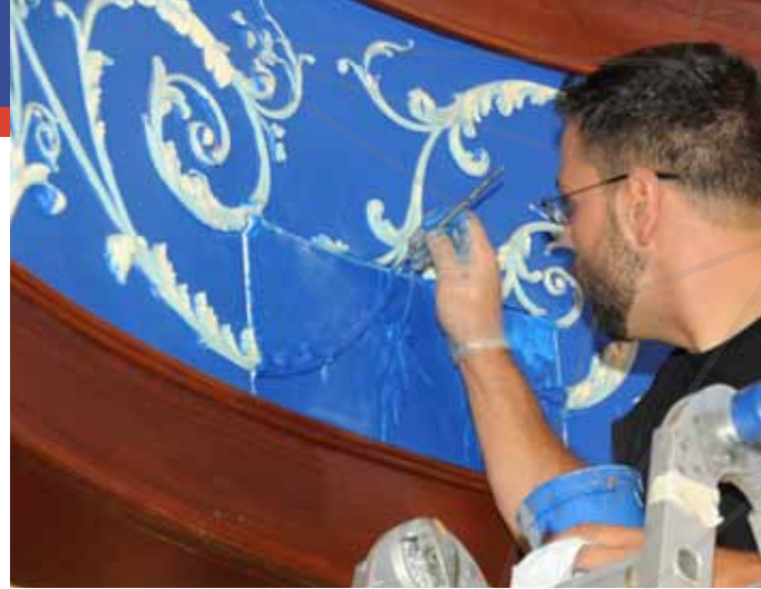
A SKILLED ARTISAN CAREFULLY REPAIRS DECORATIVE PLASTER
