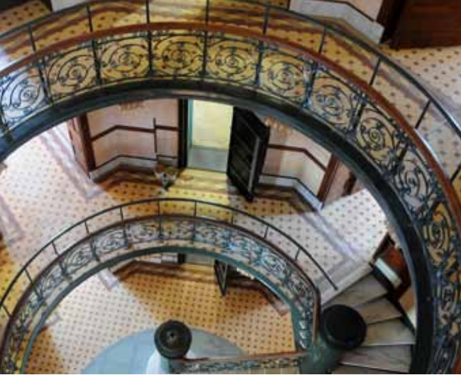
FULLY-RESTORED ORNATE RAILINGS IN THE CENTRAL STAIRCASE
